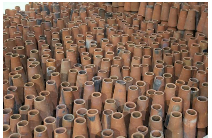
Handmade terracotta pots from Auroville were individually unwrapped to be stacked for the main barrel vault
