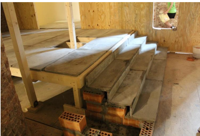
4-piece jigsaw timber around Corderie column
