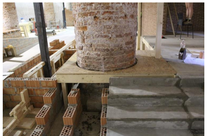
4-piece jigsaw timber around Corderie column
