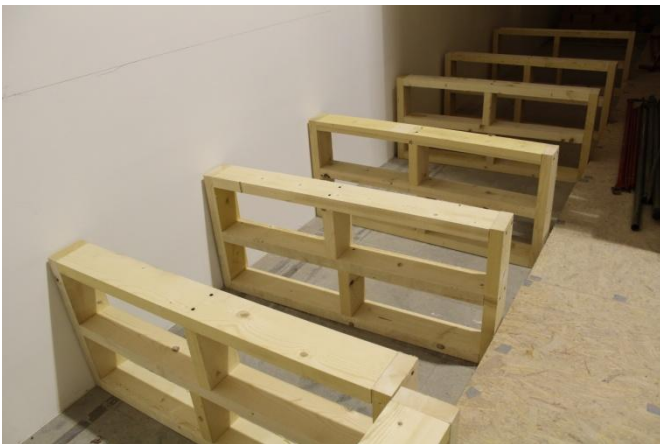
Completed timber spreader frames for new floor
