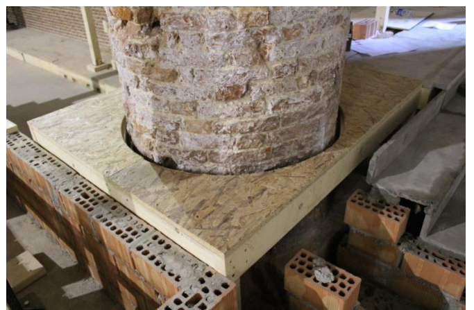
4-piece jigsaw timber around Corderie column
